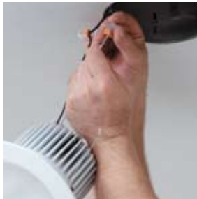
Simply remove Edison adapter from CRL6K-G2 module and insert wires into Quick Connectors on * for a high efficacy installation.
